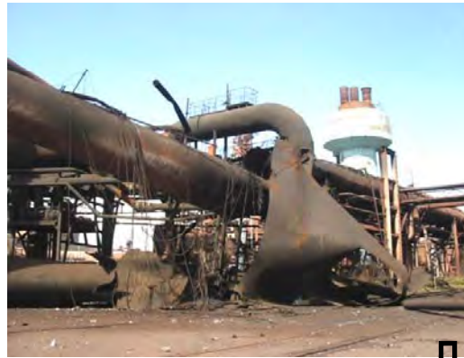
Damaged coke gas pipe
