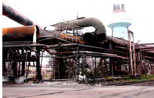
Damaged parts are being replaced.
