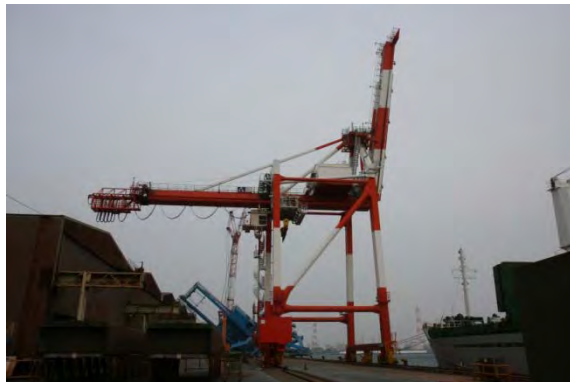
Substitute crane moved to Kashima from Wakayama steelworks
